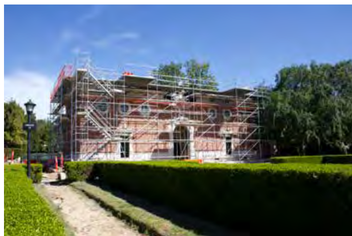
Scaffolded Clark Library and walkway, 23 March 2016
